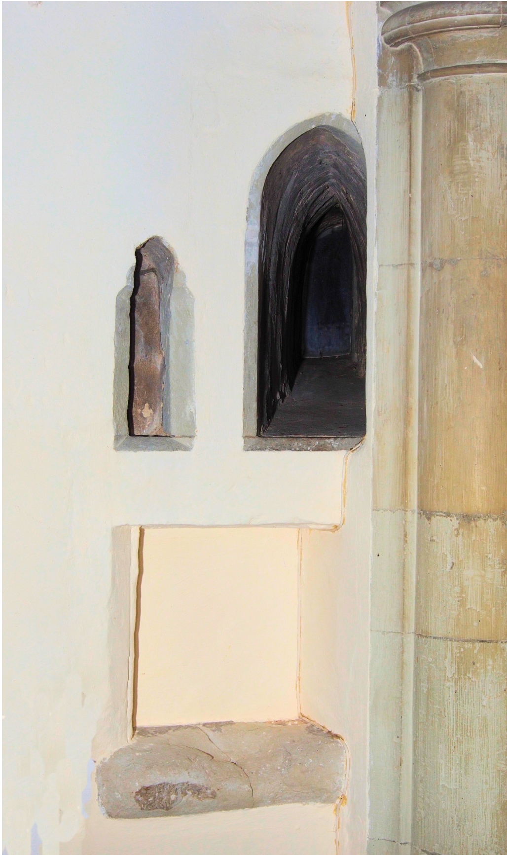
Niche top left, squint top right with piscine underneath
