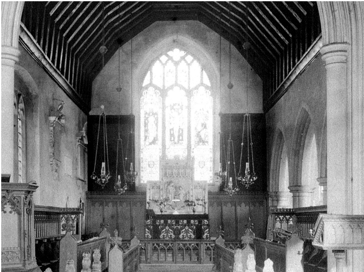
Old picture showing original reredos in place.
